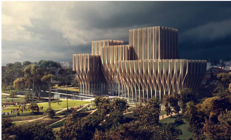
The south facade of the Sleuk Rith Institute, as designed by the architect Zaha Hadid. (Sleuk Rith Institute)
